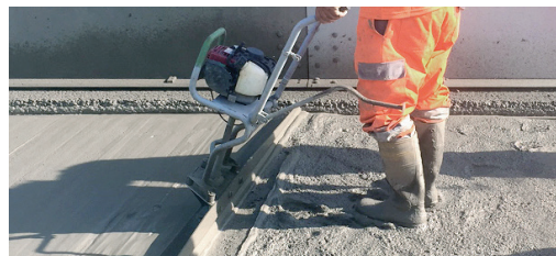
Horizontale Reprofilierung: re-bar in Sika MonoTop-452 N
