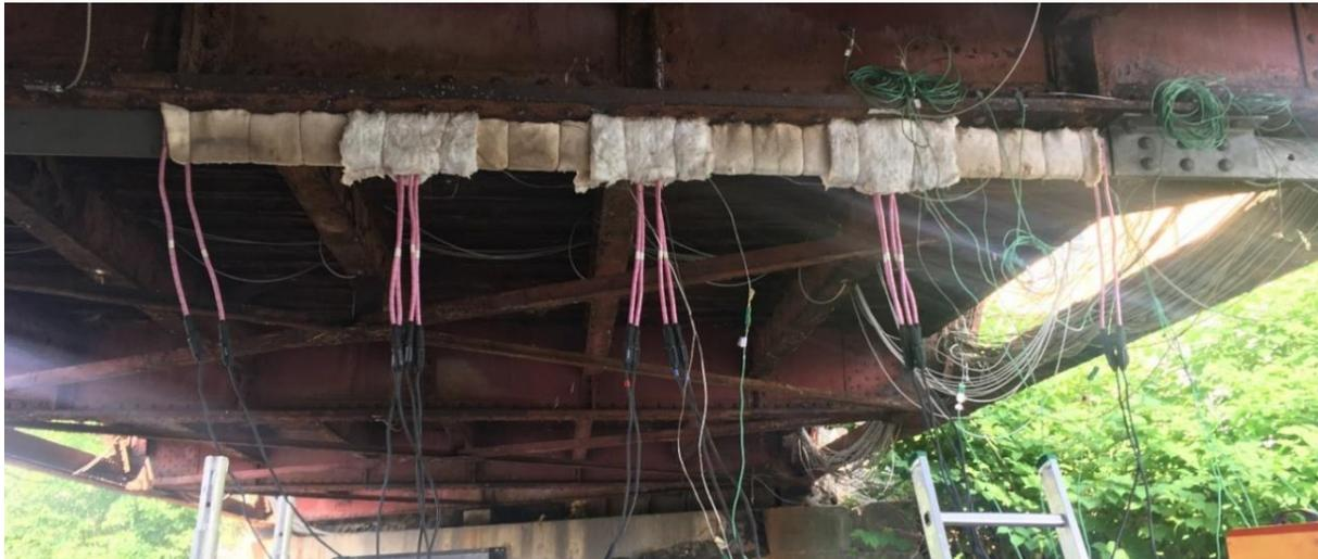
Figure 5. Heating of the second half of the Fe-SMA plates.
