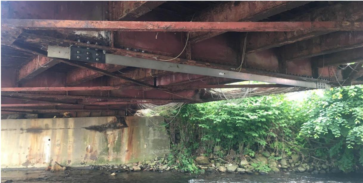
Figure 8. Final configuration of the SMA-strengthened girder of Petrov Bridge.
