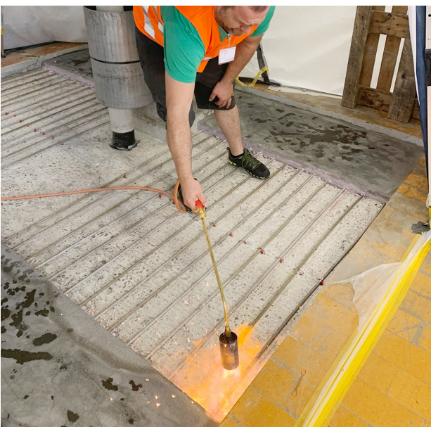
2. Activeren re-bar m.b.v. Gasbrander
