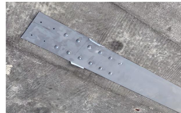
3. re-plate Zugband am Beton
