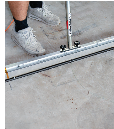
4 Activate «heating» of re-bar with re-IR 1500 infrared heater
