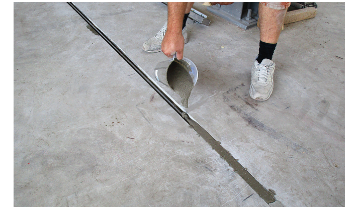
5 Filling with SikaGrout 311 between double-sided end anchors
