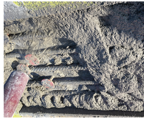
3B Double-sided embedding in Sika MonoTop-422 PCC «Sprayed mortar» as final anchoring
