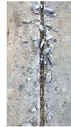
1 Slitting the concrete groove in the concrete substrate (Width 3.5 cm / depth 2.5 cm / for re-bar \text{Ø}12 \text{ mm} )
