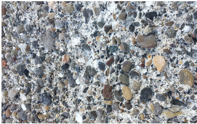
1 Hydromechanical roughening of the concrete substrate
