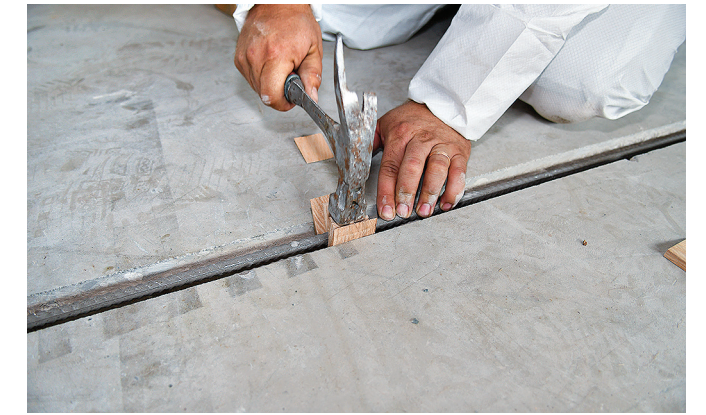
2 fixing rebar centrally in concrete groove
