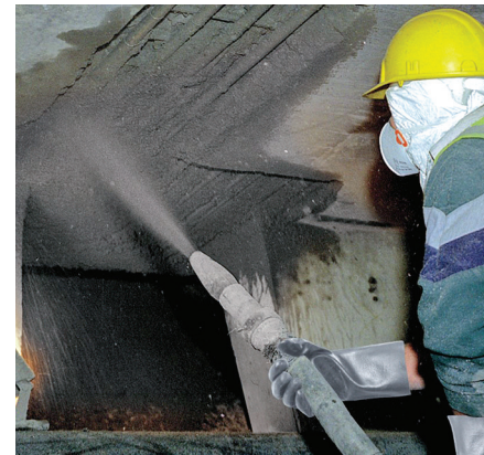
5B Apply Sika MonoTop-422 PCC between the end anchors
