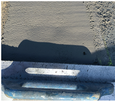
3A Double-sided embedding in Sika MonoTop-452 N «Reprofiling mortar» as final anchoring
