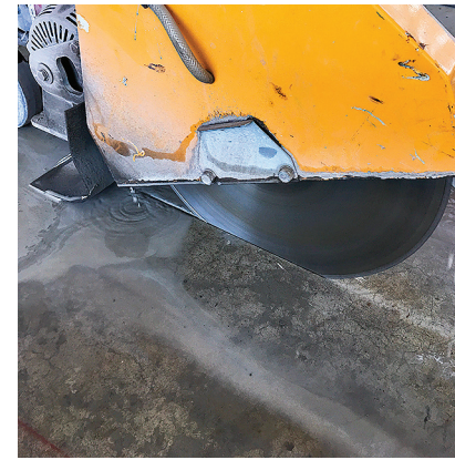
1 Slitting the concrete groove in the concrete substrate (Width 3.5 cm / depth 2.5 cm / for re-bar \text{Ø}12 \text{ mm} )
