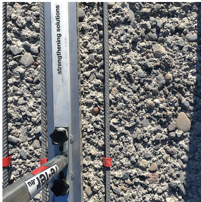
4 Activation «heating» of re-bar with re-IR 1500 infrared heater
