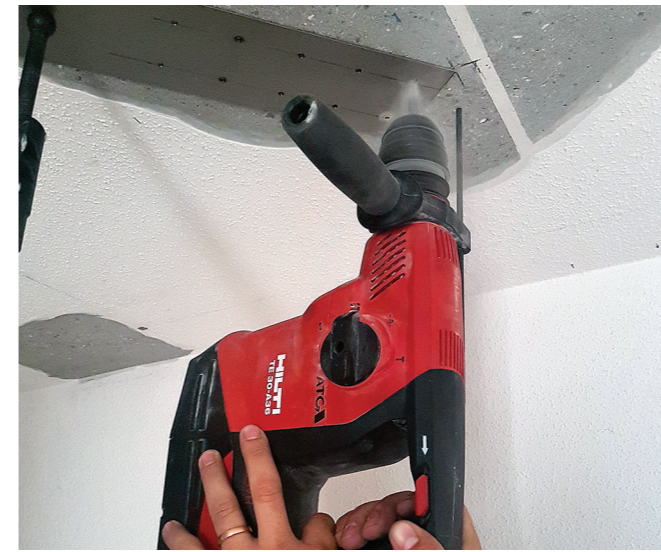
3 Pre-drill supporting surface through pre-punched re-plate \varnothing 3.5 mm
