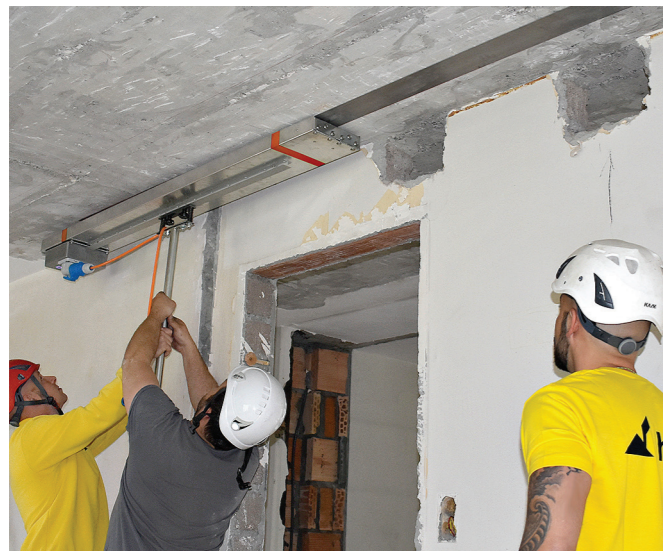
5 Step-wise heating with re-IR 3000 infrared radiant heater
