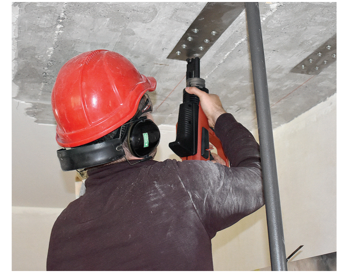
4 Mechanically end-anchoring with Hilti DX 5 powder activated tool and system-tested stainless steel nails (X-CR 48 P8 S15)
