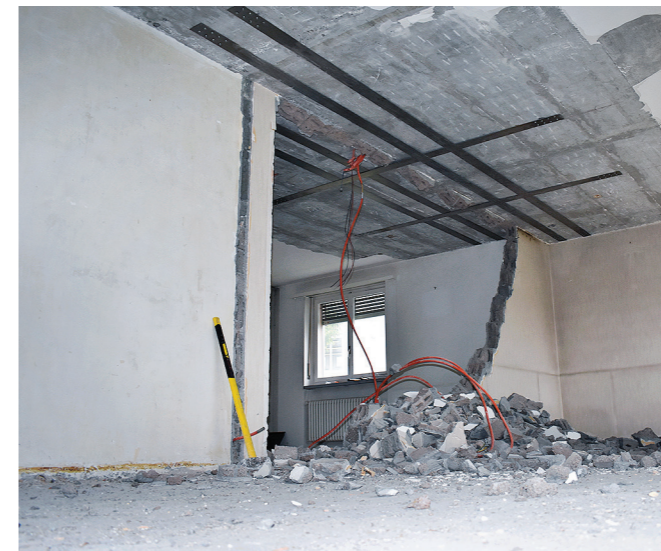
7 Applied and pre-stressed re-plate - load-bearing components can now be removed - if necessary, apply the system-tested Sika fire protection system
