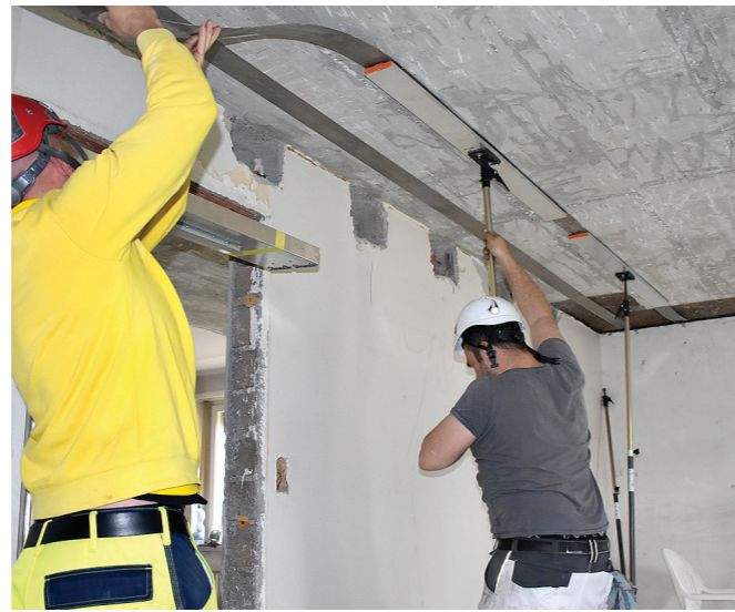
2 Temporary fixing of re-plate with T-supports
