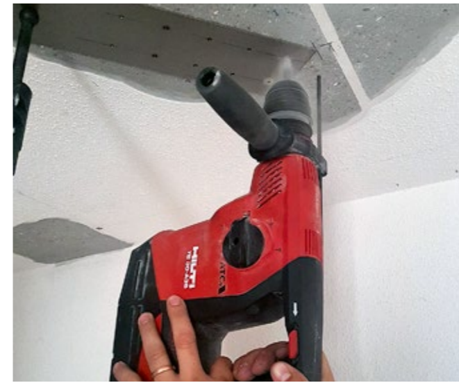
3 Pre-drill supporting surface through pre-punched re-plate Ø 3.5 mm
