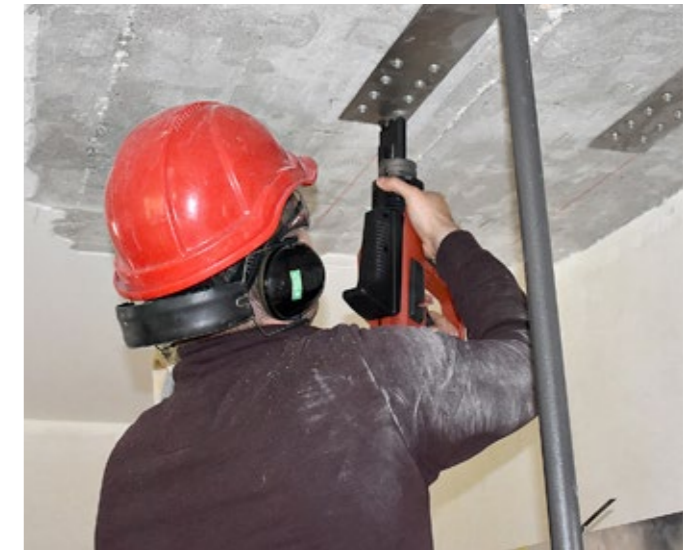
4 Mechanically end-anchoring with Hilti DX 5 powder activated tool and system-tested stainless steel nails (X-CR 48 P8 S15)
