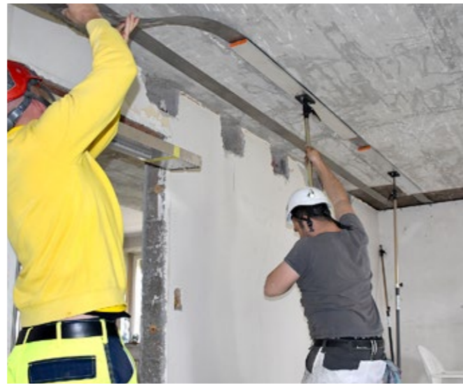
2 Temporary fixing of re-plate with T-supports
