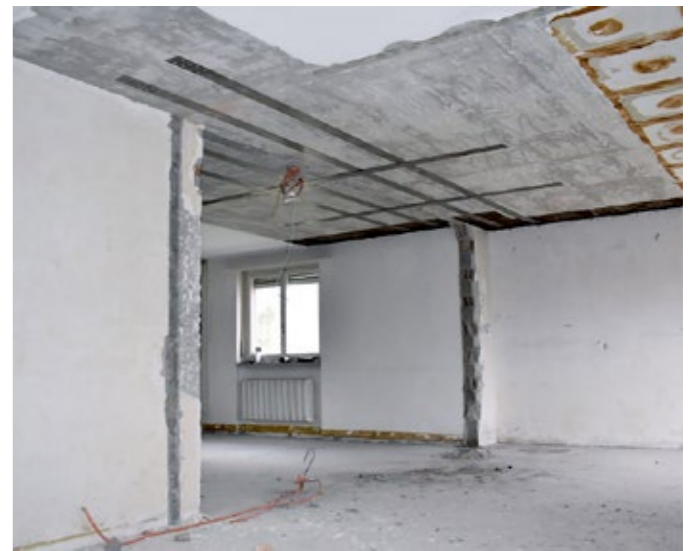
7 Applied and pre-stressed re-plate - load-bearing components can now be removed - if necessary, apply the system-tested Sika fire protection system
