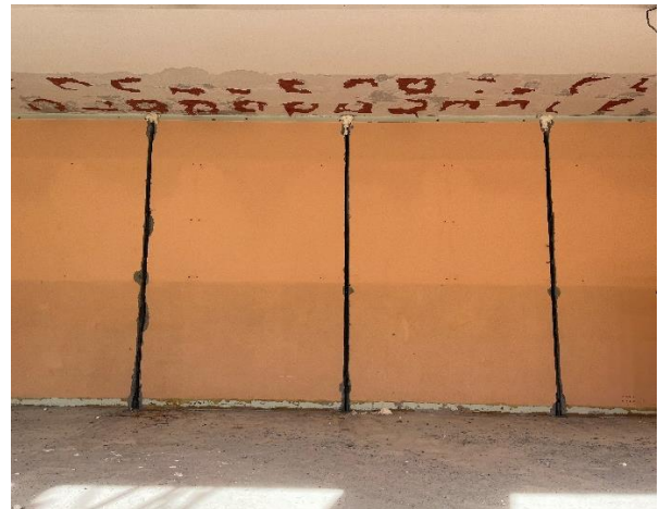
Cut grooves with anchored re-bars
