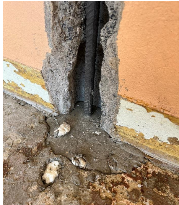
Mortar anchoring of re-bar in floor slab
