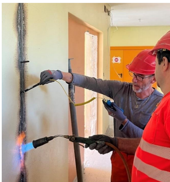
Heating of the bars and temperature control
