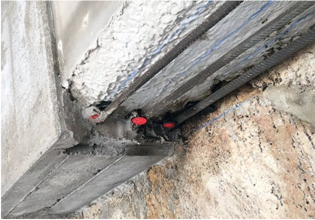
Anchoring zone of three re-bar 16 (prestressed) with three U-stirrups Ø12 mm (conventional reinforcing steel) in Sika sprayed mortar
