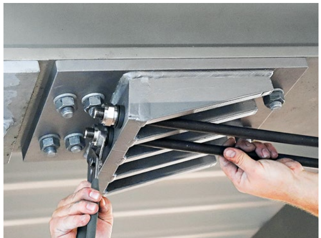
Fastening of end anchorage
