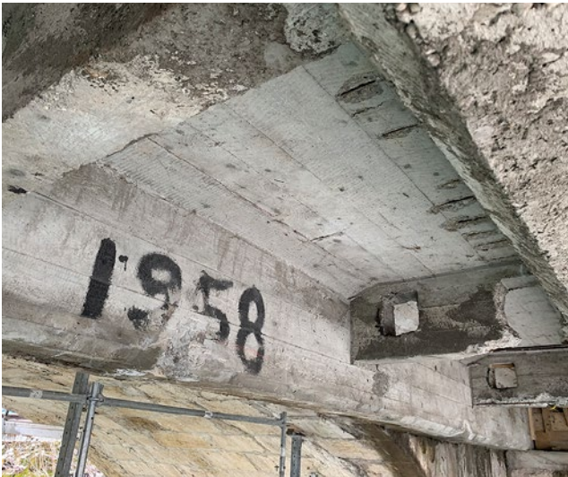
Poor quality concrete before retrofitting
