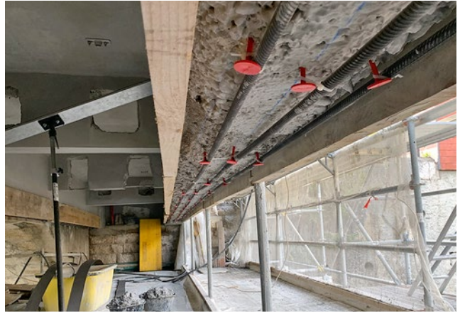
Anchoring zone of three re-bar 16 (prestressed) with three U-stirrups Ø12 mm (conventional reinforcing steel) in Sika sprayed mortar
