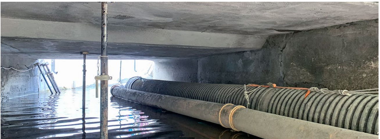
Improved flow in the culvert under the bridge after strengthening
