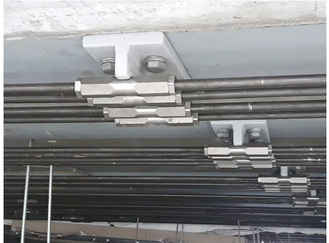
Intermediate supports in the centre of the beams
