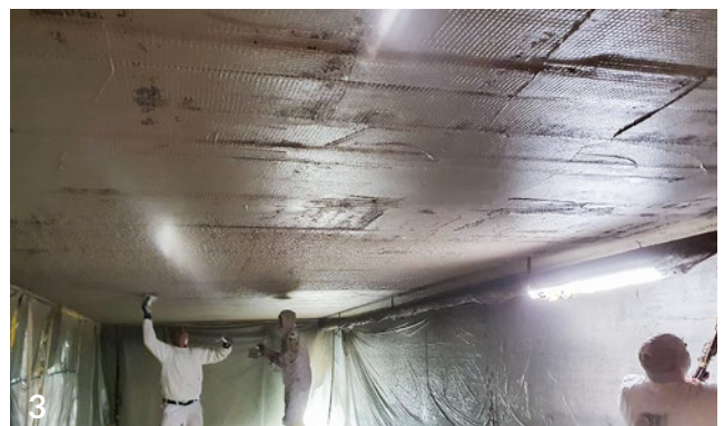
Fire protection for re-plate in combination with CFR strip
