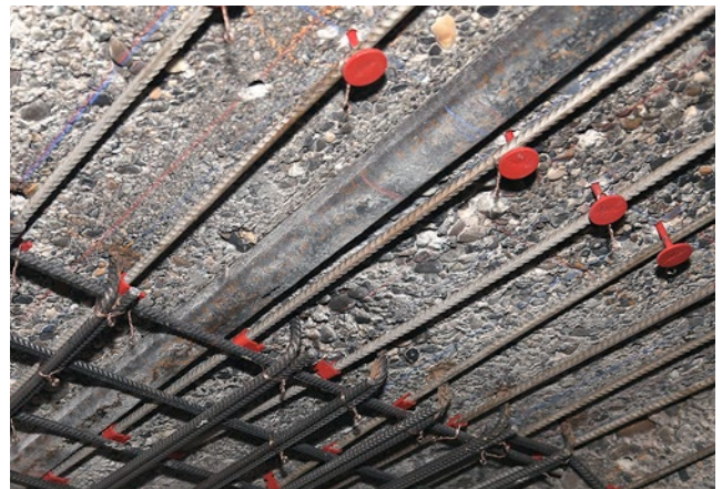
Fixing the re-bar to internal reinforcement (with re-clip) and to the concrete substrate (with re-bolt)
