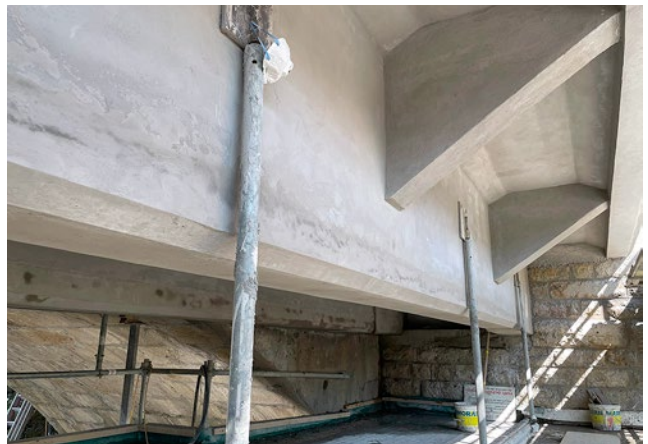
After strengthening: Finishing Sika mortar on the complete surface
