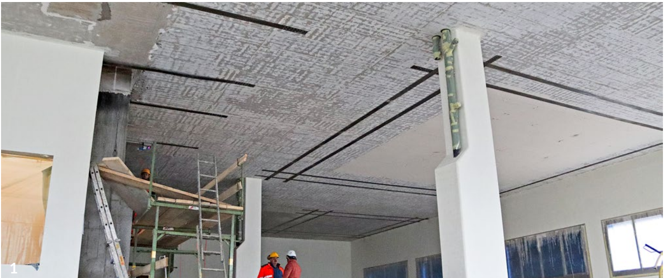
Typical strengthening of the positive bending moment with re-plate
