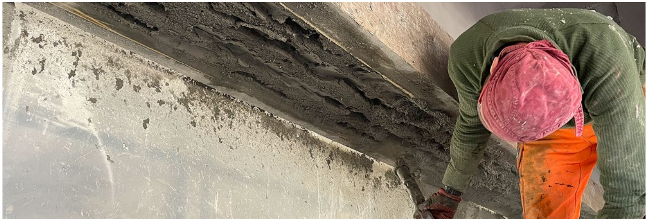
Embedding re-bar in Sika sprayed mortar
