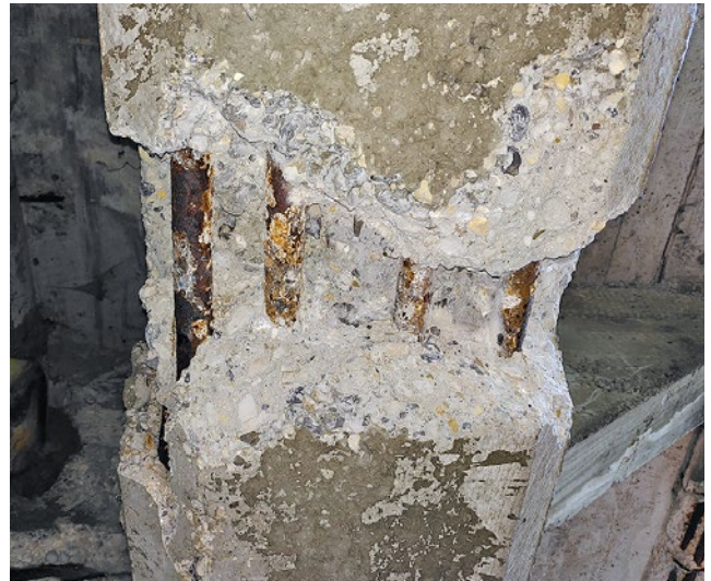
Corroded internal reinforcement
